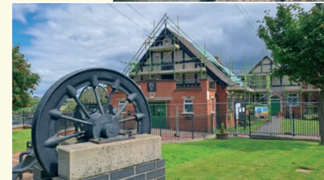
Work on Great Houghton Miners' Welfare Hall.
