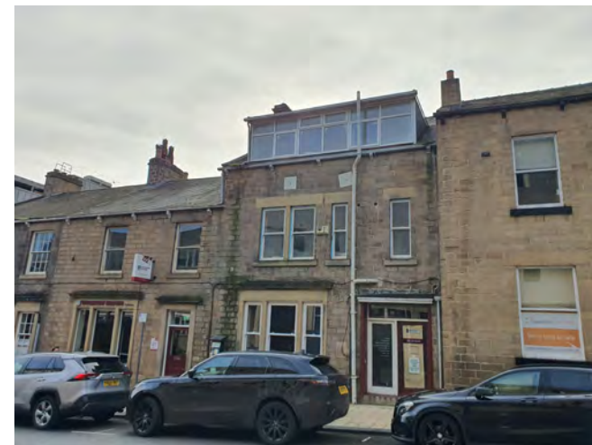
Inappropriate full-width roof dormer
