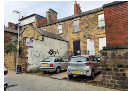
Loss of rear boundary wall to allow car parking to the rear of Regent Street
