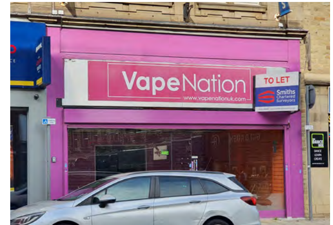
Vacant shop on Eldon Street
