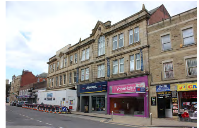
Former YMCA and Eldon Buildings
