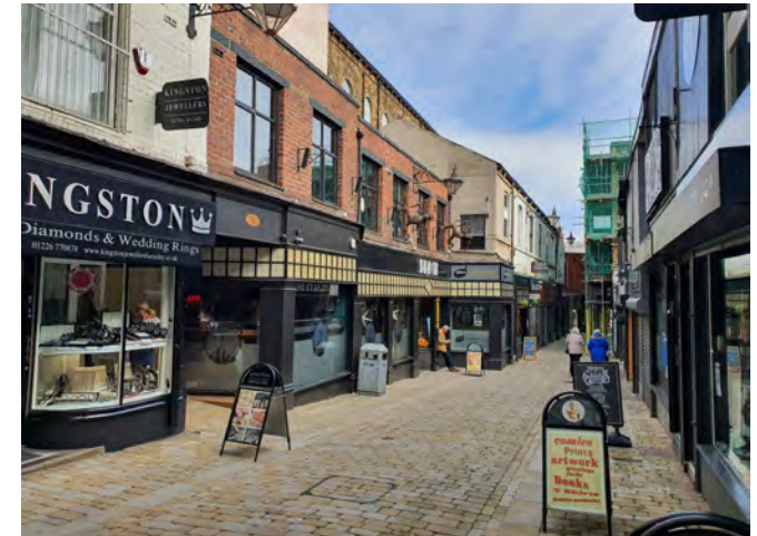
Eastern end of the Arcade
