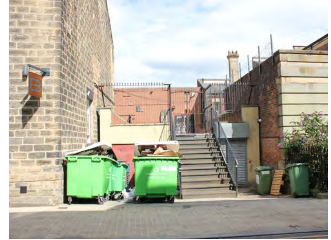
Views of the rear of buildings and bins from the public realm mar the visitor experience in a number of areas. This example is in Eastgate.
