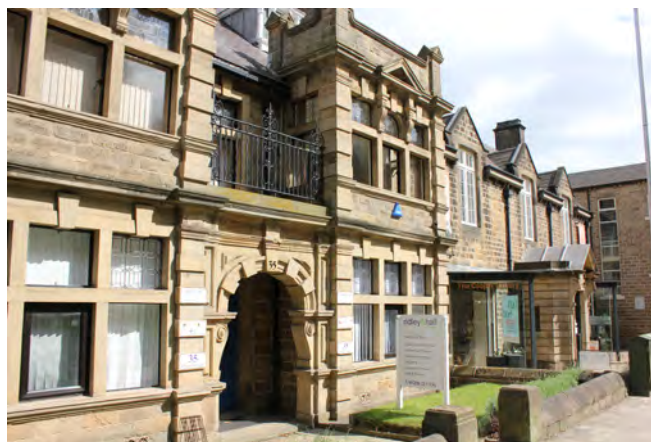
Buildings maintained in a good state of repair
