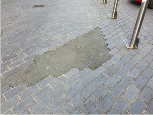
Patched repairs of a recently paved surface, now requiring a more appropriate repair
