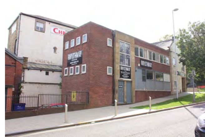
Modern building to rear of Church Street
