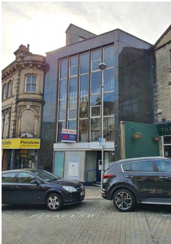
Vacant unit on Market Hill
