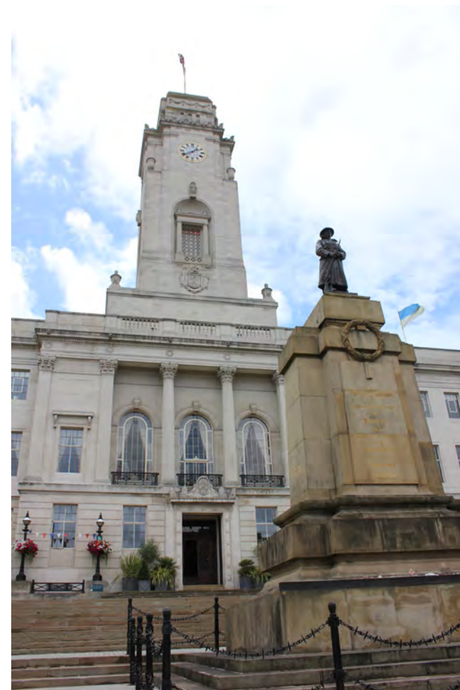
Town Hall and attached railings are listed Grade II, whilst the war memorial is Grade II*
