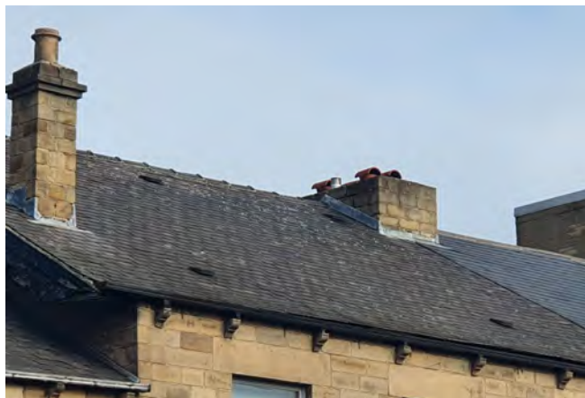
Partial removal of chimney in Regent Street
