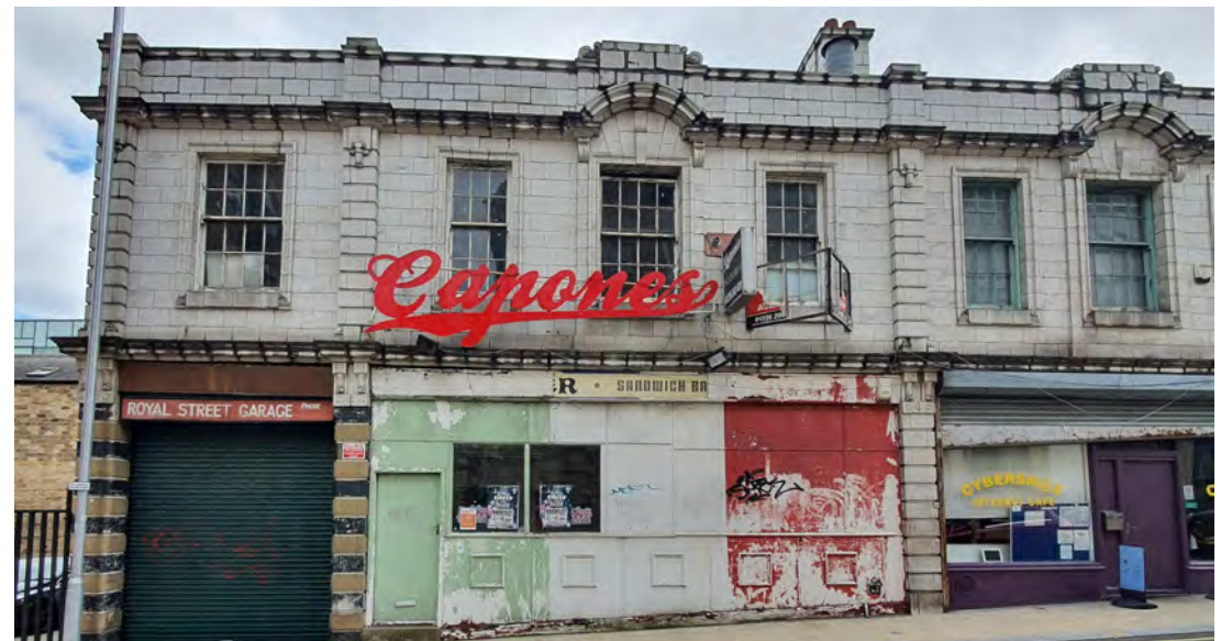
Vacant garage and restaurant, Royal Street
