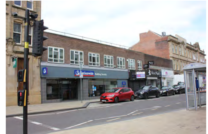
Less-than sympathetic later twentieth century intrusion on Eldon Street
