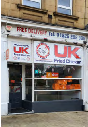
Cheaply produced and overlarge signage obscures this otherwise traditional shopfront
