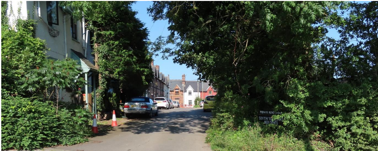
South Yorkshire Buildings, Silkstone Common
