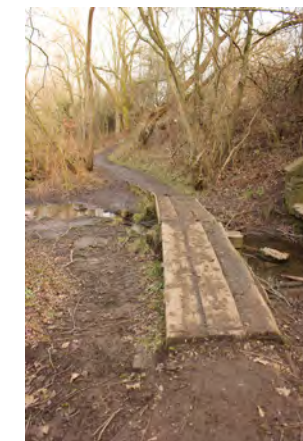
Footpaths could be improved around the reservoir
