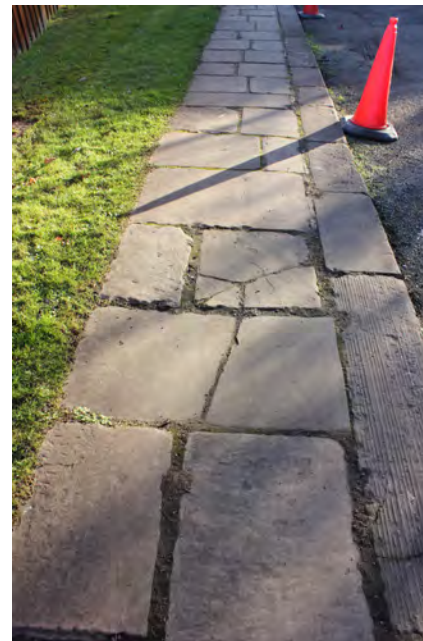
Stone flags and stone kerbs
