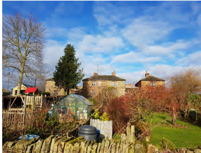
Grade II listed Skiers Hall Cottages
