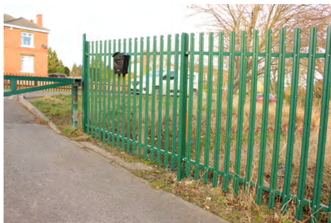
Intrusive security fencing
