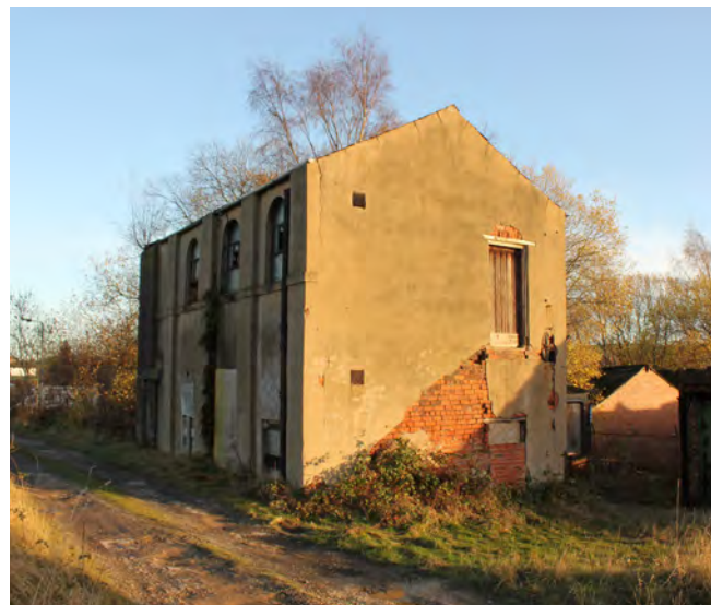
Davy Iron Foundry buildings
