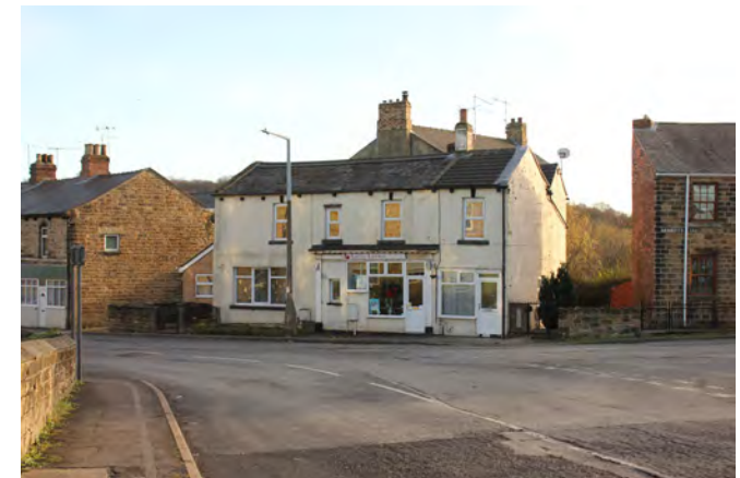
Rendered stone building also in need of maintenance
