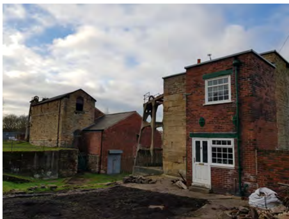
Former pump house (left) and Engine House (right), Hemingfield Colliery
