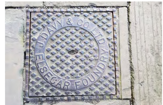
Manhole cover from the Davy Foundry
