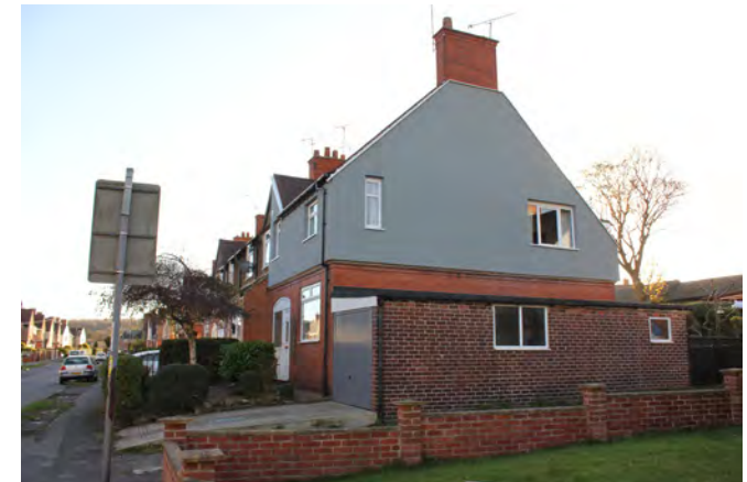
External cladding and garage extension, Trafford Avenue
