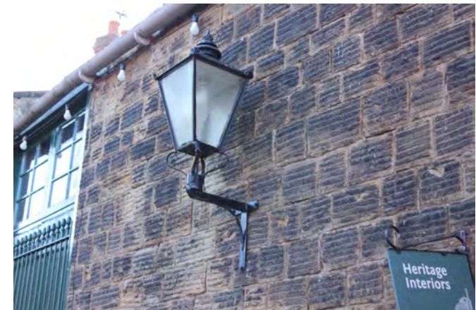
Lantern on Building 4
