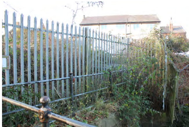
Modern fencing beside the canal basin
