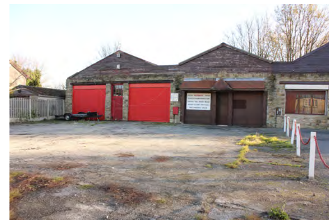
Vacant former garage on Wath Road
