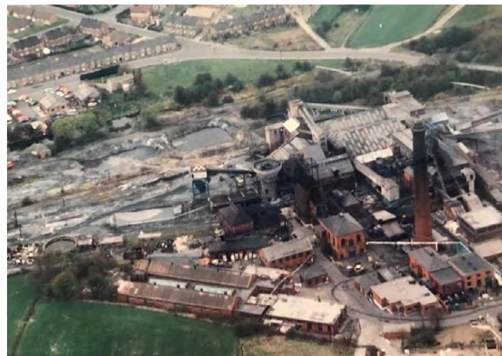
Aerial view of Elsecar Main before closure
