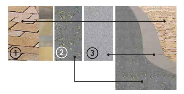
There is flexibility in the placement of the wide flush yorkstone kerb, which can be laid either centrally or in a traditional street pattern. Drainage design should align with kerb lines to avoid additional detailing.
