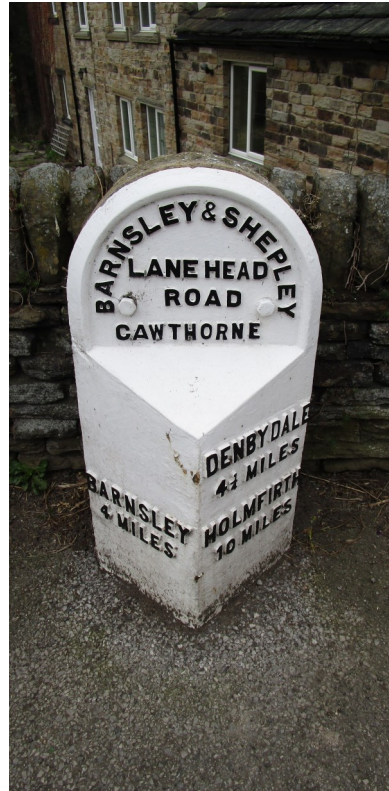
Plate 47: Grade II listed milestone, Hill Top
