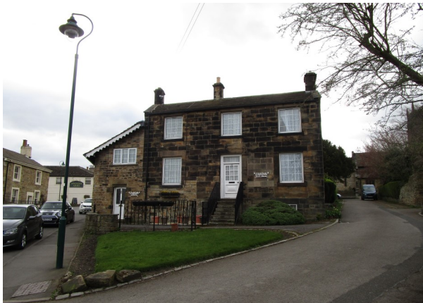
Plates 49 and 50: UPVC doors and windows replace historic features and undermine the character and appearance of the conservation area
