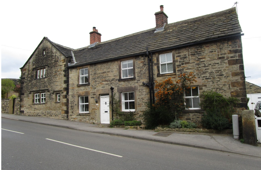
Plate 35: Nos. 31 and 33 Darton Road
