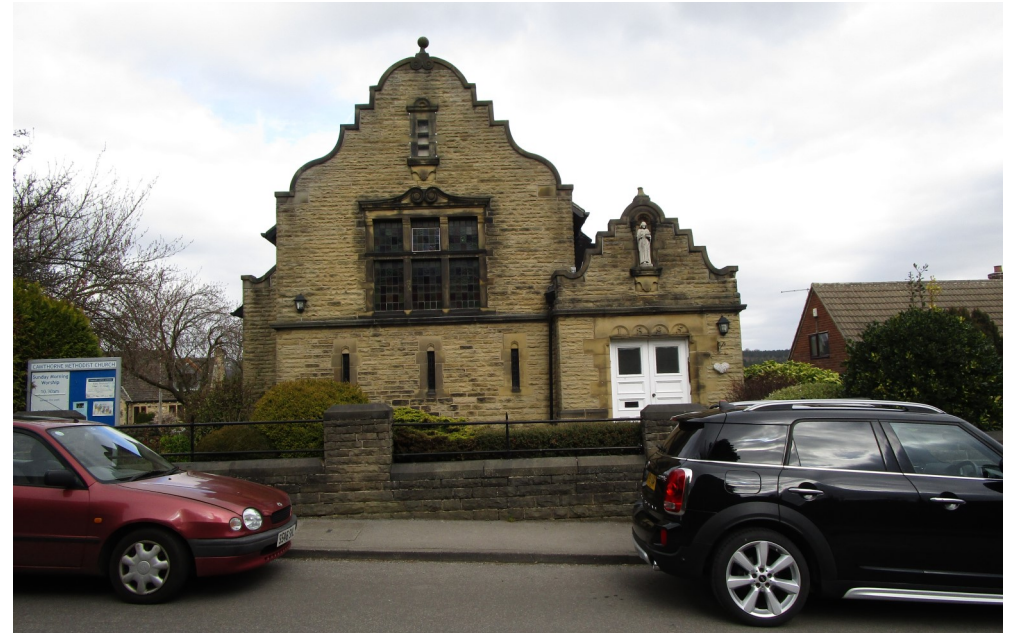
Plate 10: Cawthorne Methodist Church, Darton Road
