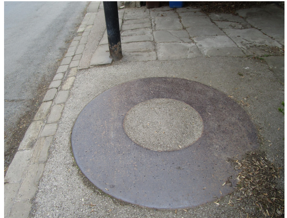
Plate 48: Wheel mould in pavement outside No. 2 Tivy Dale (former smithy)
