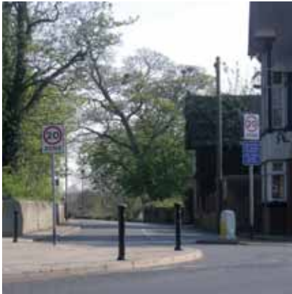
Footway build-outs can be an effective means of speed reduction on existing streets
