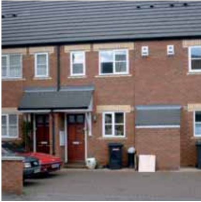
Standard, small terraced house types do not perform well in meeting Code for Sustainable Homes standards, in particular for storage of waste and recycling and access to rear gardens
