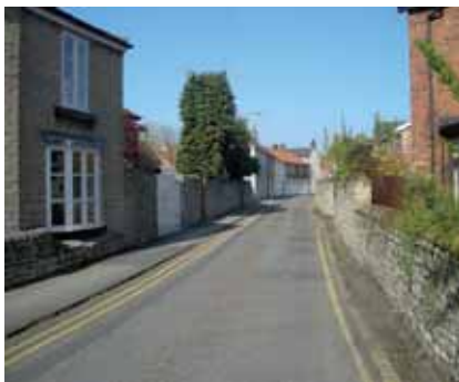
The ratio for this street is about 1:1.5, and gives an intimate feel suited to shorter lanes and links
