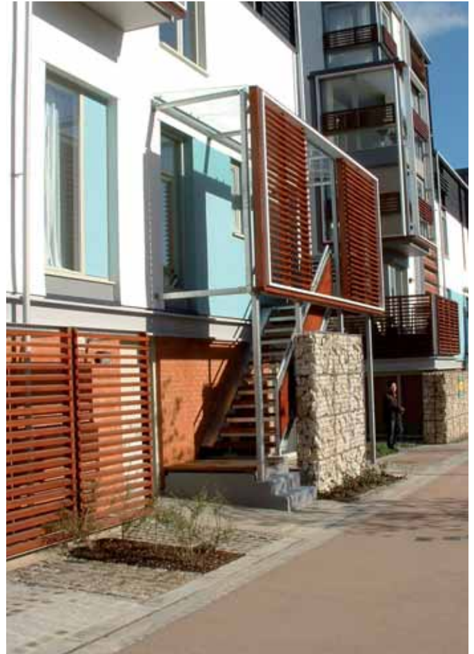
The transition space at the entrance gives a balance between privacy and an active frontage (the stair is a secondary entrance)
