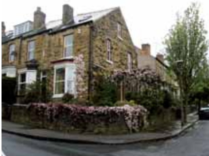
This end terrace in Crookes, Sheffield turns the corner with a door and windows on the gable end
