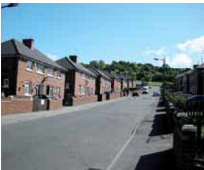
An example of mid-20th century development at Bessacar, Doncaster
