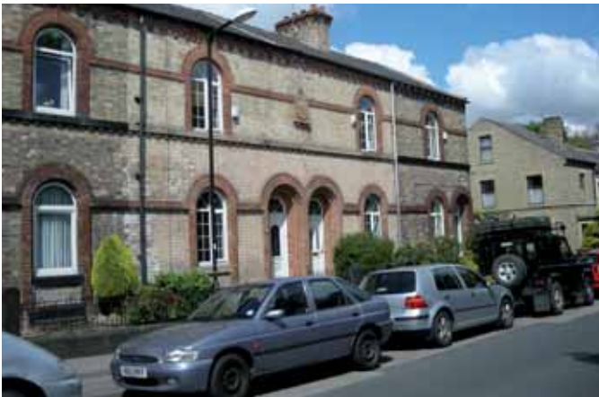
The combination of active openings and more elaborate detail in Old Town, Barnsley, create a strong public front to the building
