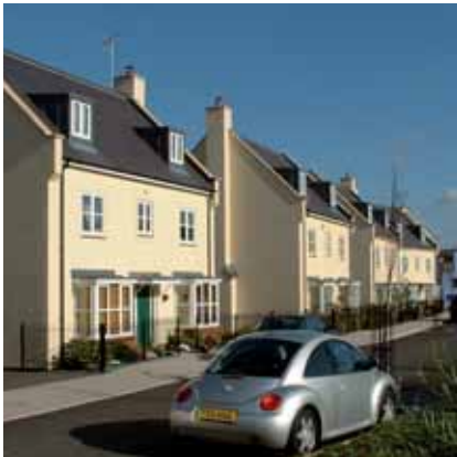
On-street parking within a widened carriageway
