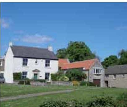
The basic building types in South Yorkshire are relatively simple in form and for that reason are versatile in how they can be adapted to new standards
