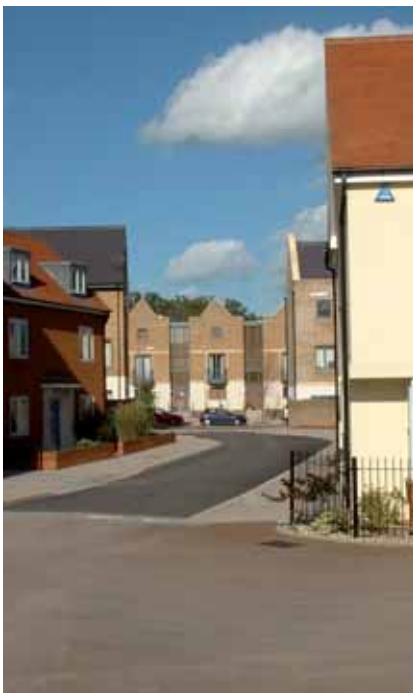
The raised table junction in the foreground combined with good enclosure creates a general feel that higher speeds are inappropriate (other features may be necessary in some situations to define the protected zone)
