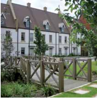
SuDS schemes can be an integral part of the street scene that gives it its character
